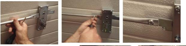
4. Fit the keeper plate onto the channel using the two M6 screws provided.
