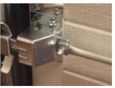
2. Fit the operating bar on to the lock, lay it next to the latch and mark the end level with the edge of the latch.
