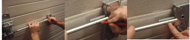
3. Cut the operating bar, flatten and drill the end. Bolt on to the latch. Check its operation
